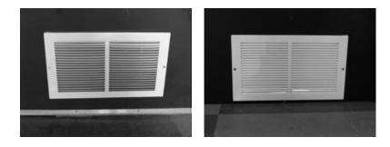
When the flow is limited or inaccessible between rooms downstairs (if there are walls or partitions), then install a grille 8" x 10" (or other grill configuration, having total area of not less than 80 sq. in.) in the bottom of the door or wall to avoid having stagnant air in those areas. Otherwise interior doors must remain open. This insures that all the air drawn into the Humidex comes from all areas of the basement.
